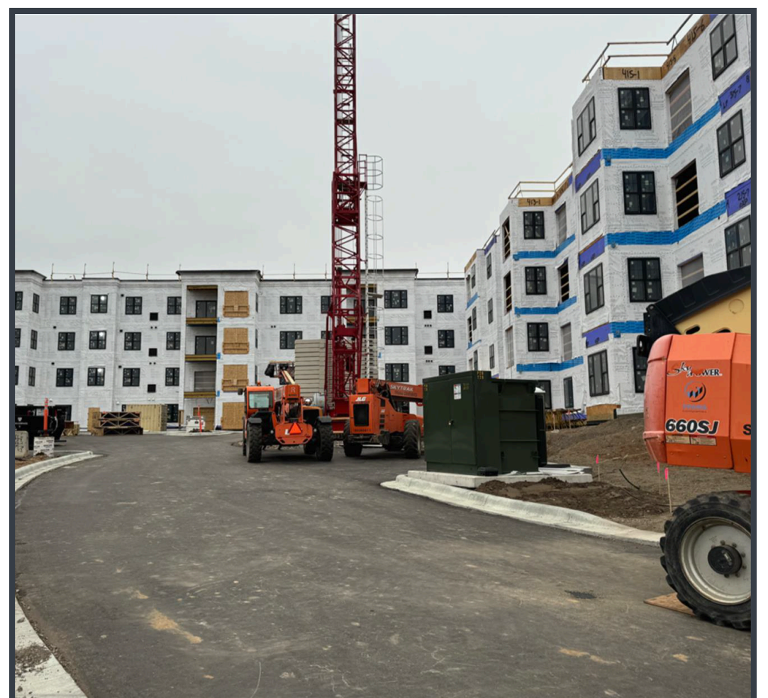
View facing north - curb and 1st layer of asphalt complete!
