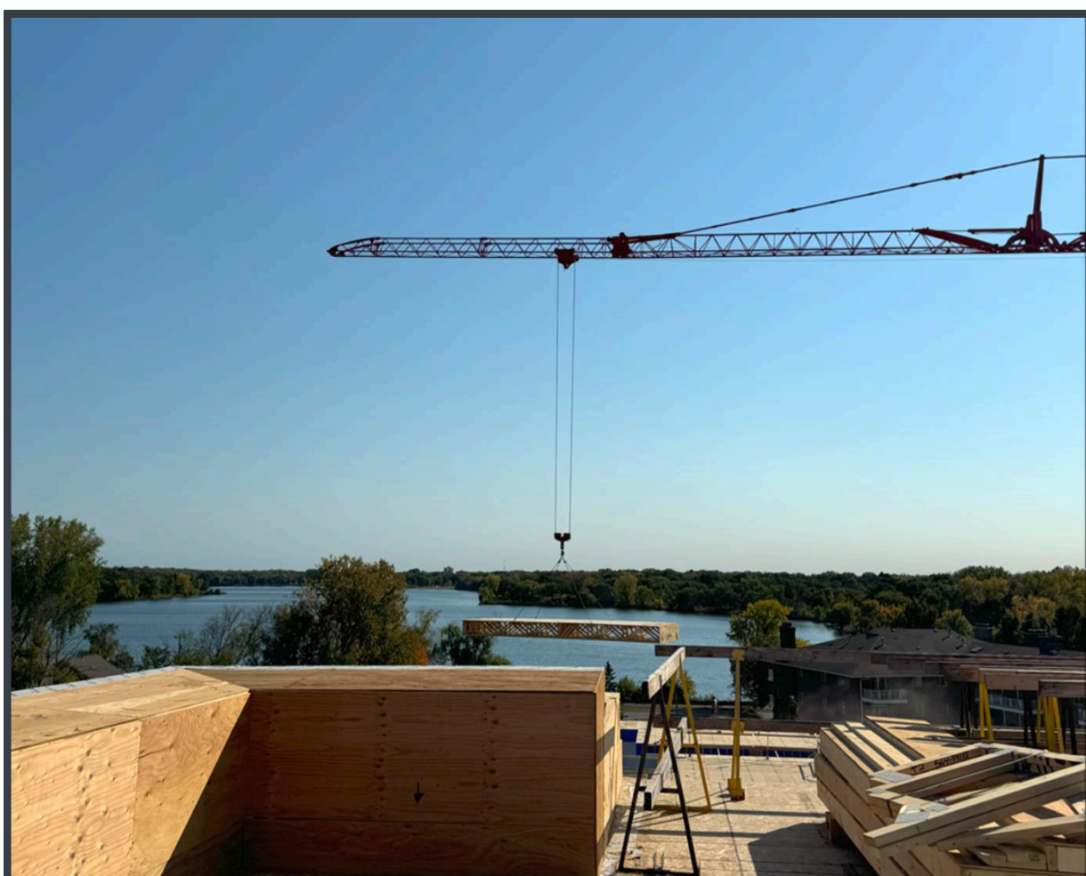
View of beautiful Lake Phalen as crane drops trusses into place.
