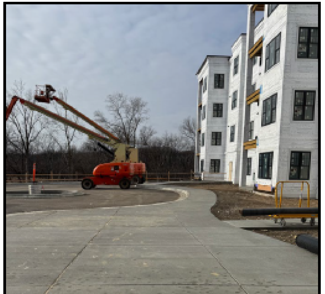
View from main entry - sidewalks complete!
