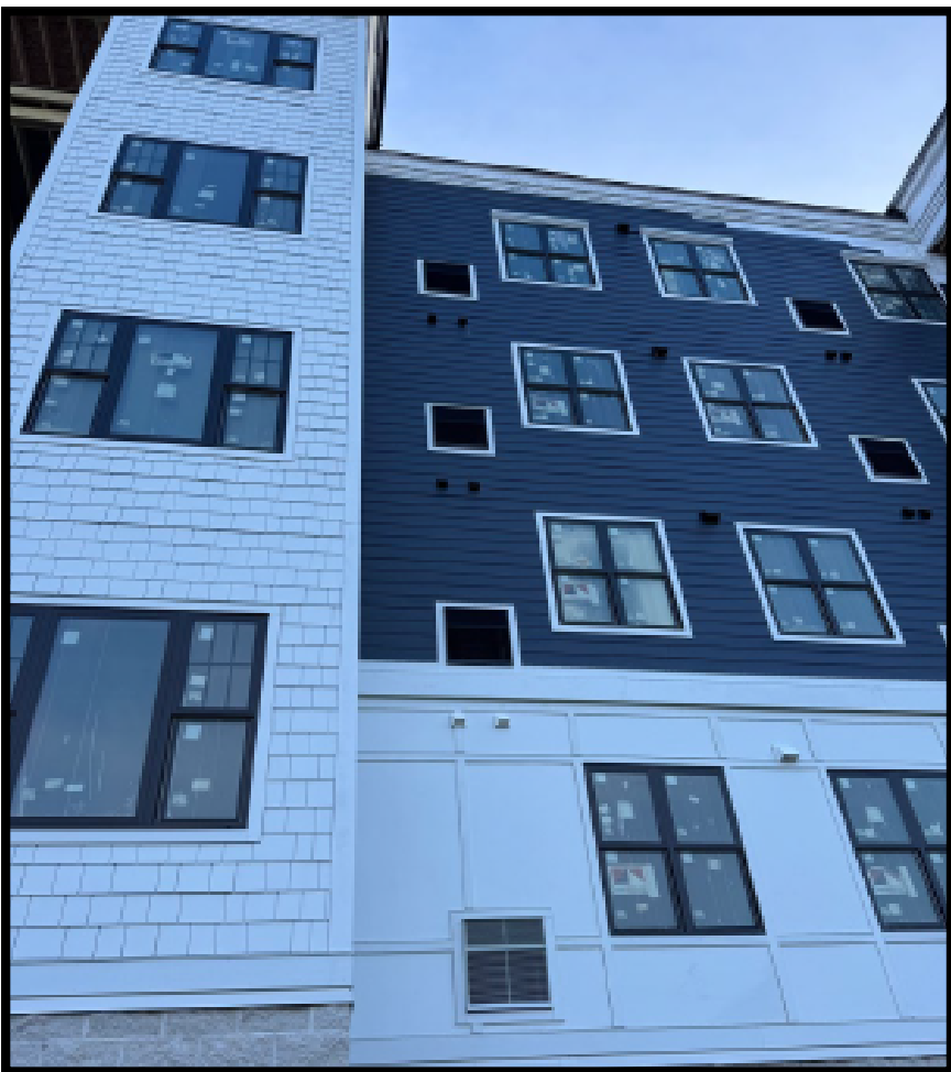
View of North elevation - siding underway!
