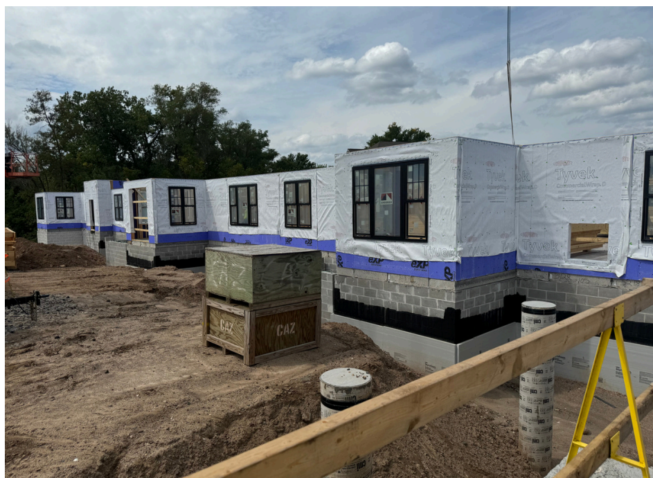
Zone 1 exterior walls & windows
