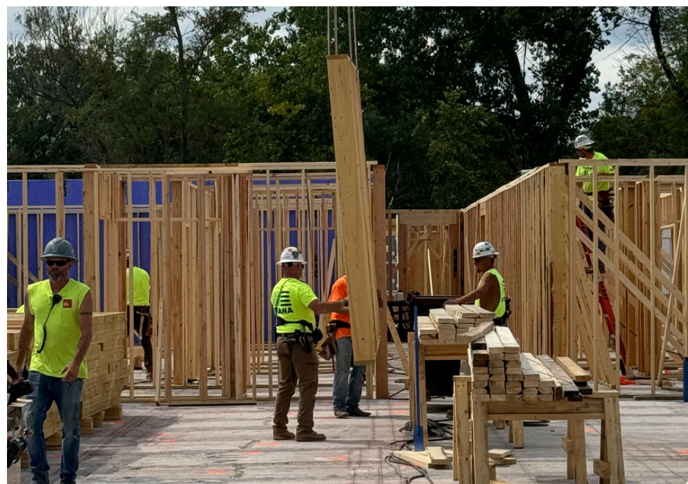
Setting a corridor wall in place
